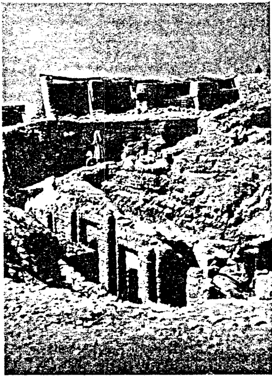
FIG. 16. VIEW OF THE FAÇADE OF THE TOMB OF NEB-AMEN.
